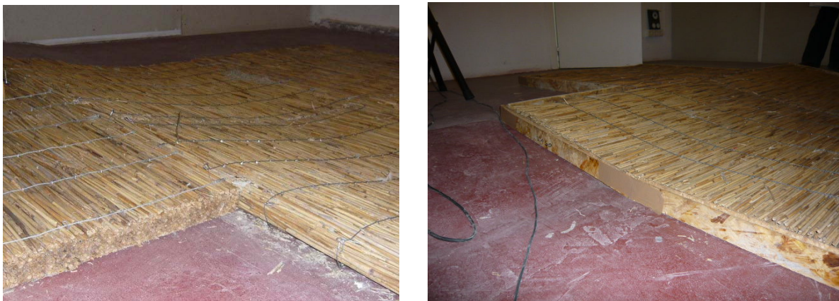
fig. 1 "Placing of reed panels on the floor"
