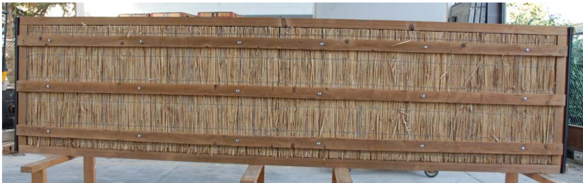
Figure 1: Picture of the noise barrier in construction for the A22 motorway near Vienna.
