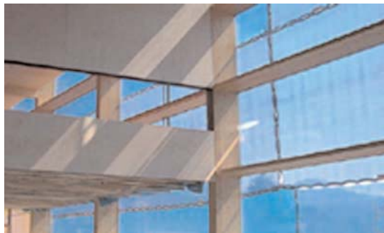
Schoolbuilding, secondary modern school, Vorarlberg
